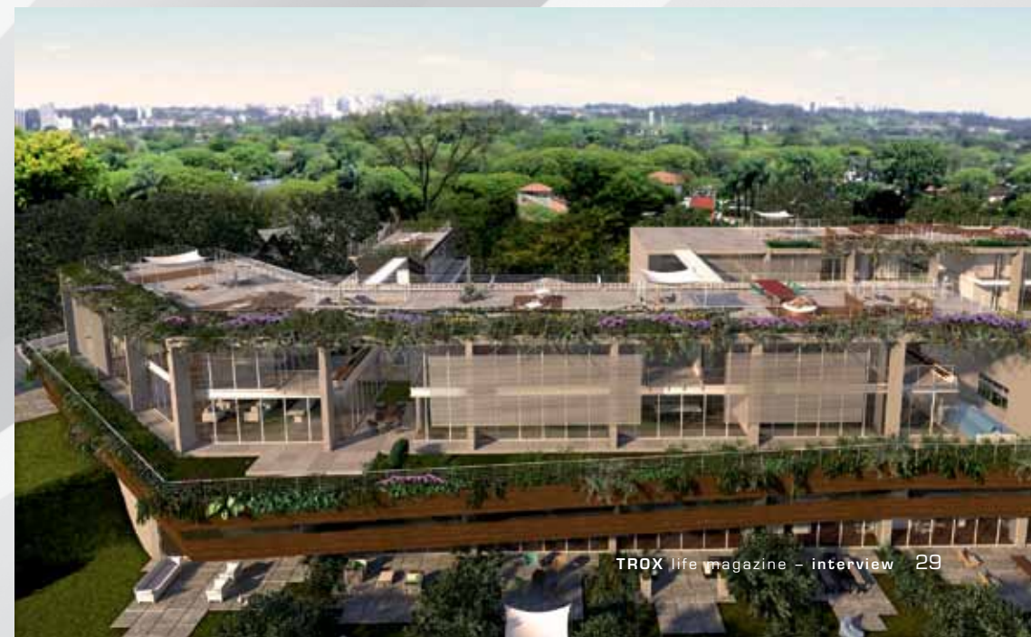
FGMF's Edificio Corujas project epitomises a triad philosophy of harmonious integration, quality of usage, and sustainability.
