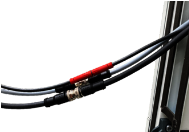
Fig. 33: Connection of the cables
