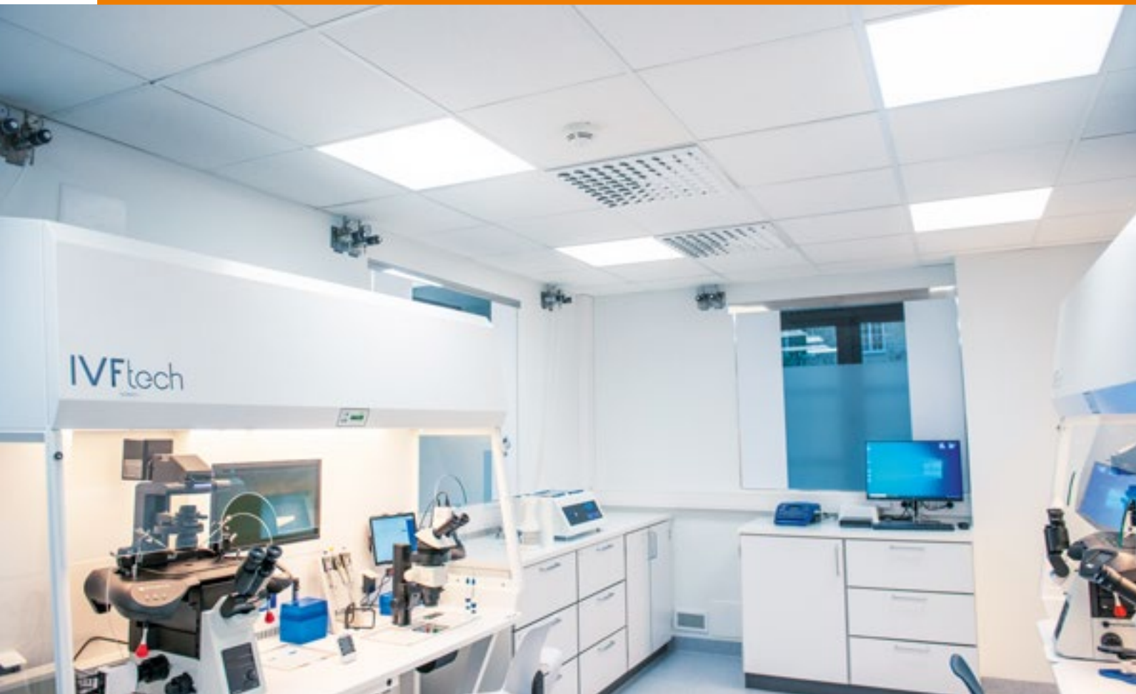
TFC ceiling mounted particulate filter with Opus diffuser face and H14 particulate filter in laboratories, examination rooms and freezer rooms.
