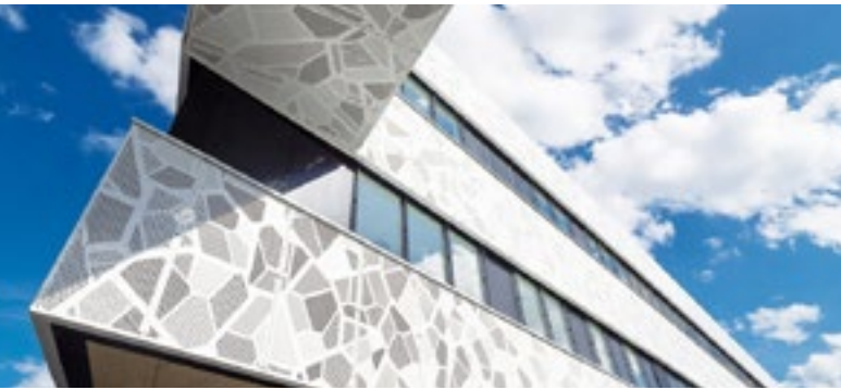
The laboratory building's air conditioning and ventilation system offers hygienic air treatment with reduced energy consumption.
