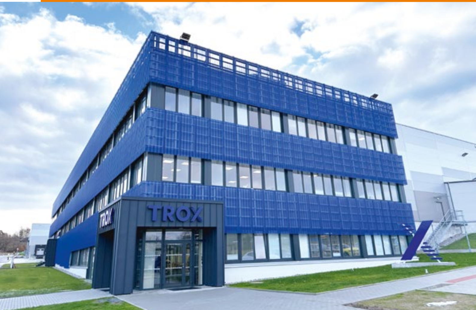
The new KS Filter production facility in the Czech Republic.
