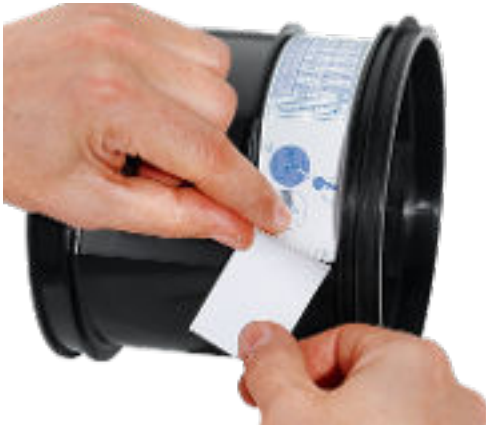
Fig. 10: Cover the slotted hole
