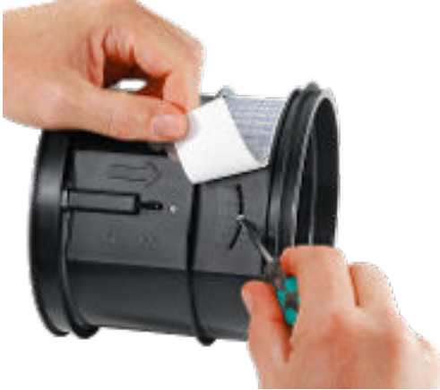
Fig. 9: Setting the volume flow setpoint
