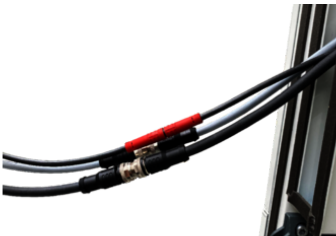
Fig. 38: Connection of the cables
