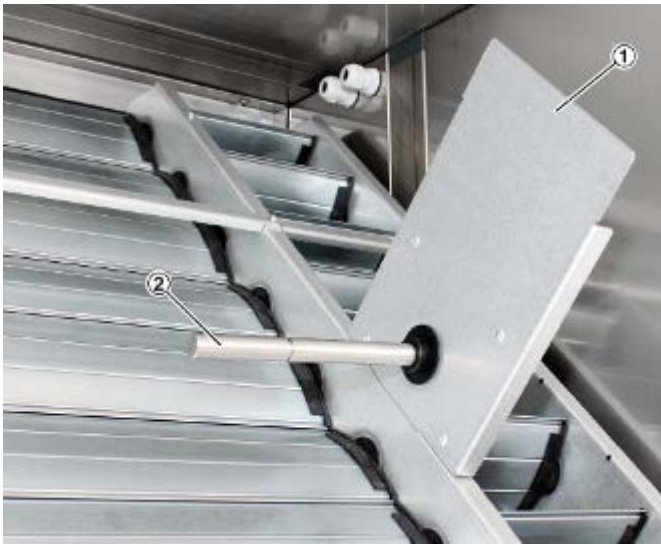
Fig. 19: H adapter with horizontal drive shaft
