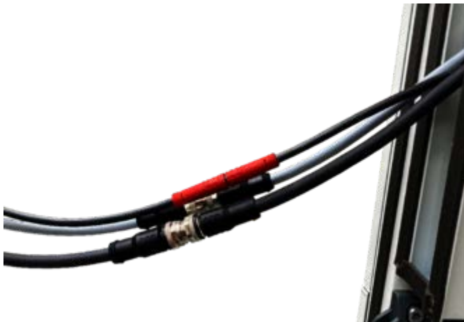
Fig. 40: Connection of the cables
